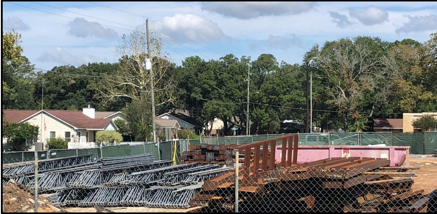
Structural Steel and Bar Joist
