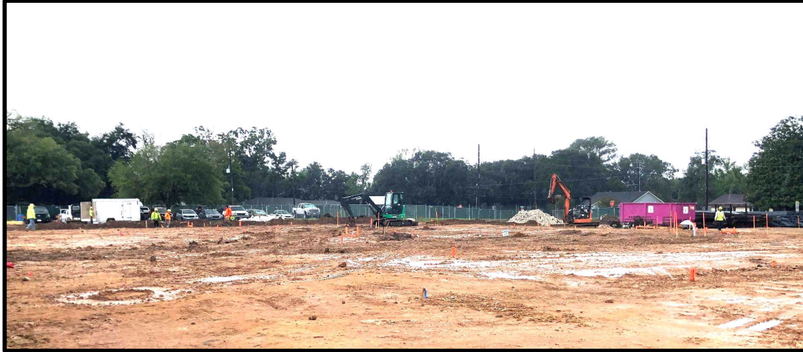
Building Pad and Grade Beams
